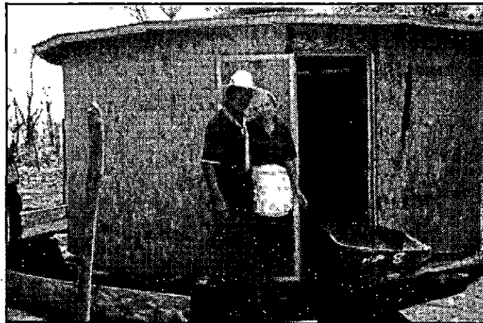
Juan and Angelica Santos stand in front of their newly built roundhouse in Rio Roldan, El Salvador.
